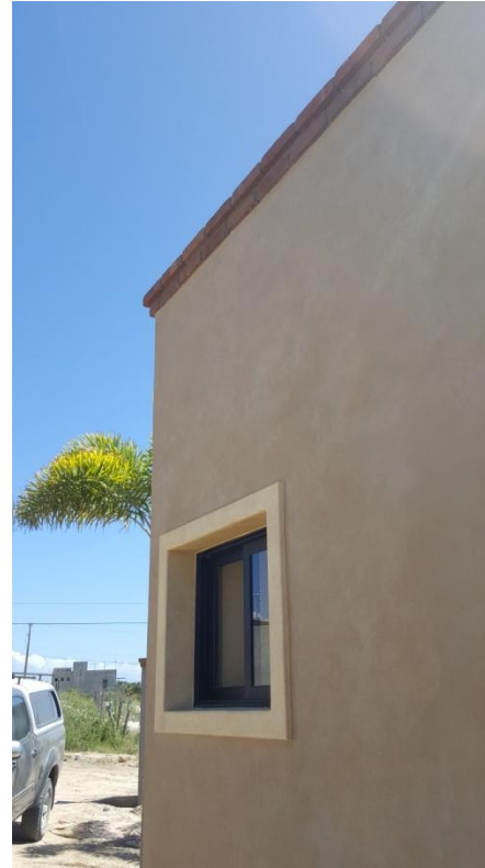
Brick Facades and Trim
